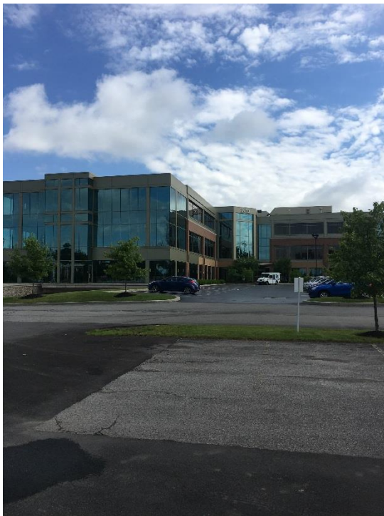
Figure 7-13. View of office park on Audubon Parkway south of I-990 (Suburban Office/Residential District)
