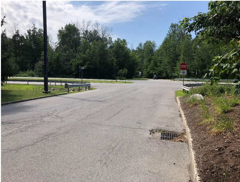
Figure 7-14. View west on Partridge Run at Audubon Parkway (Suburban Office/Residential District)
