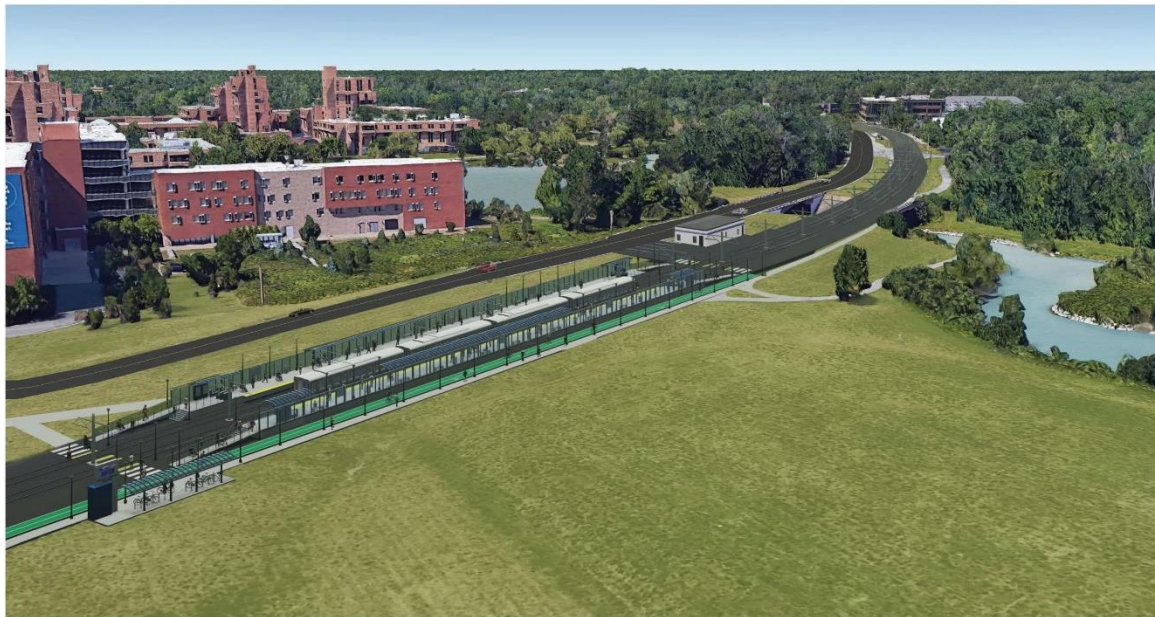
Figure 7-24. Visual Elements: Ellicott Complex Station
