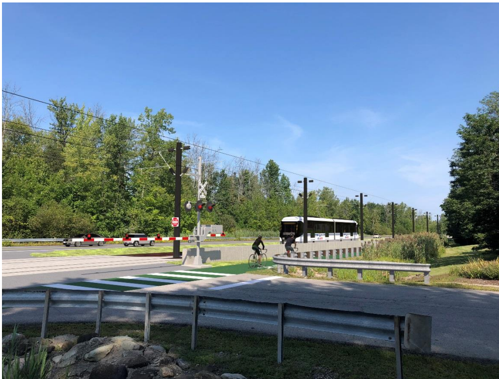
Note: This visualization is representative of conceptual design. Final selection of site details will be refined during preliminary and final design.
