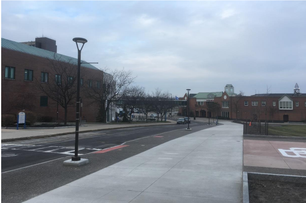
Figure 7-11. View northwest on Putnam Way adjacent to UB Student Union (University District 2)
