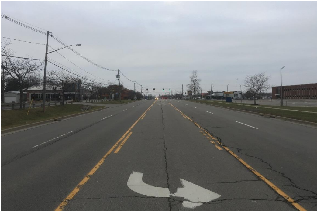
Figure 7-7. View west on Maple Road between Hillcrest Drive and Sweet Home Road (Suburban Commercial District)
