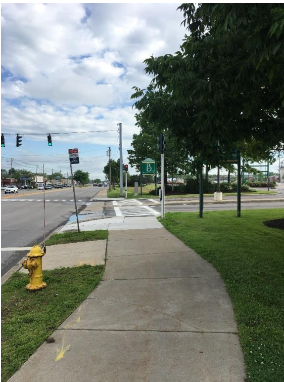
Sidewalk: Niagara Falls Boulevard
