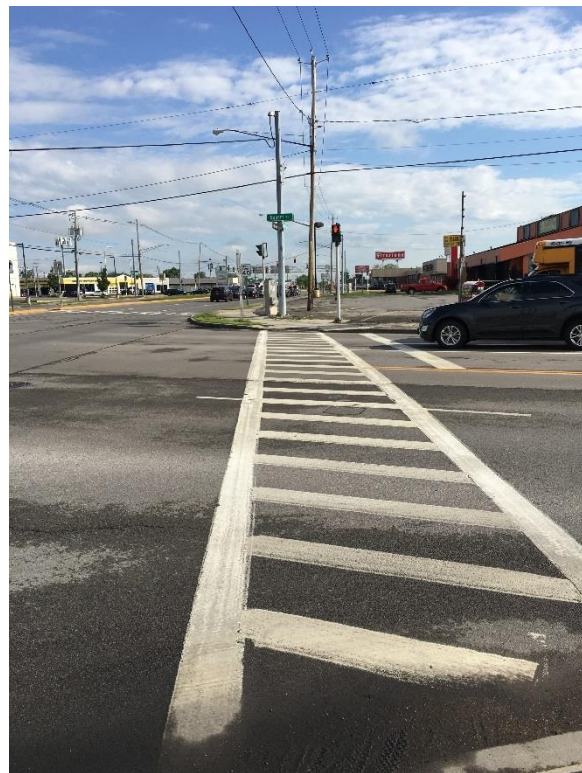
Crosswalk: Niagara Falls Boulevard and Sheridan Drive
